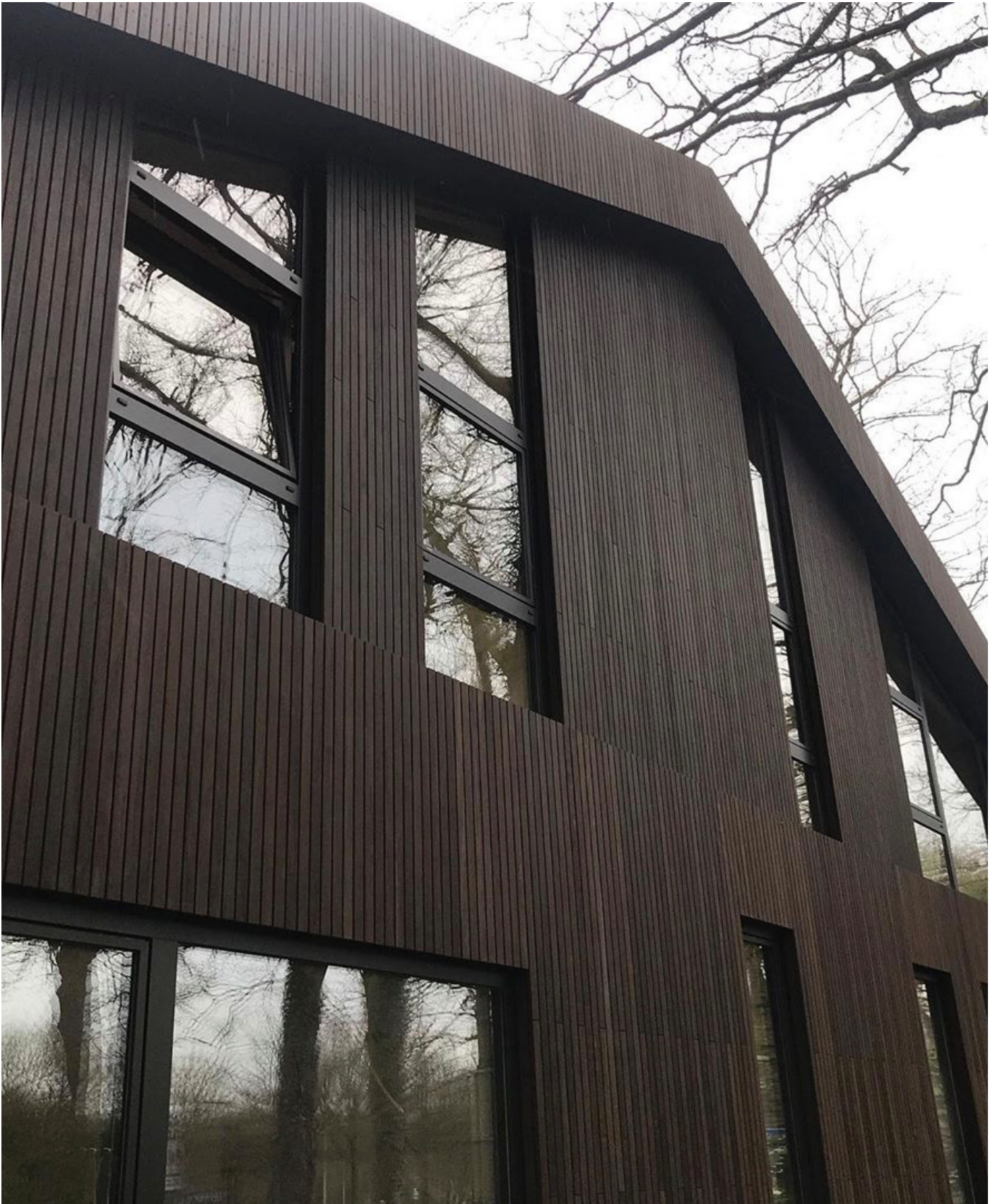
Bamboo / The Netherlands / Architect: Spee Architecten / Contractor: Awood
